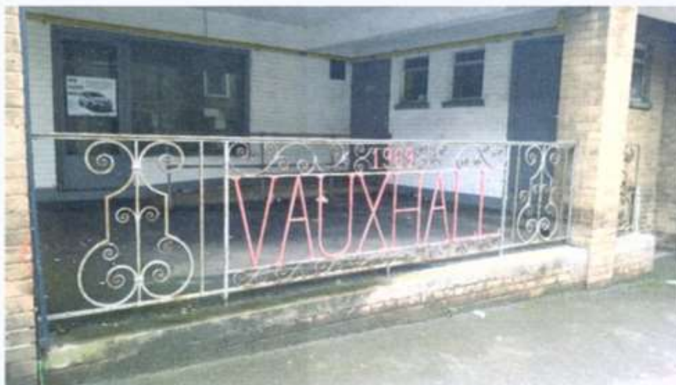
The Vauxhall Railings in the Causeway
